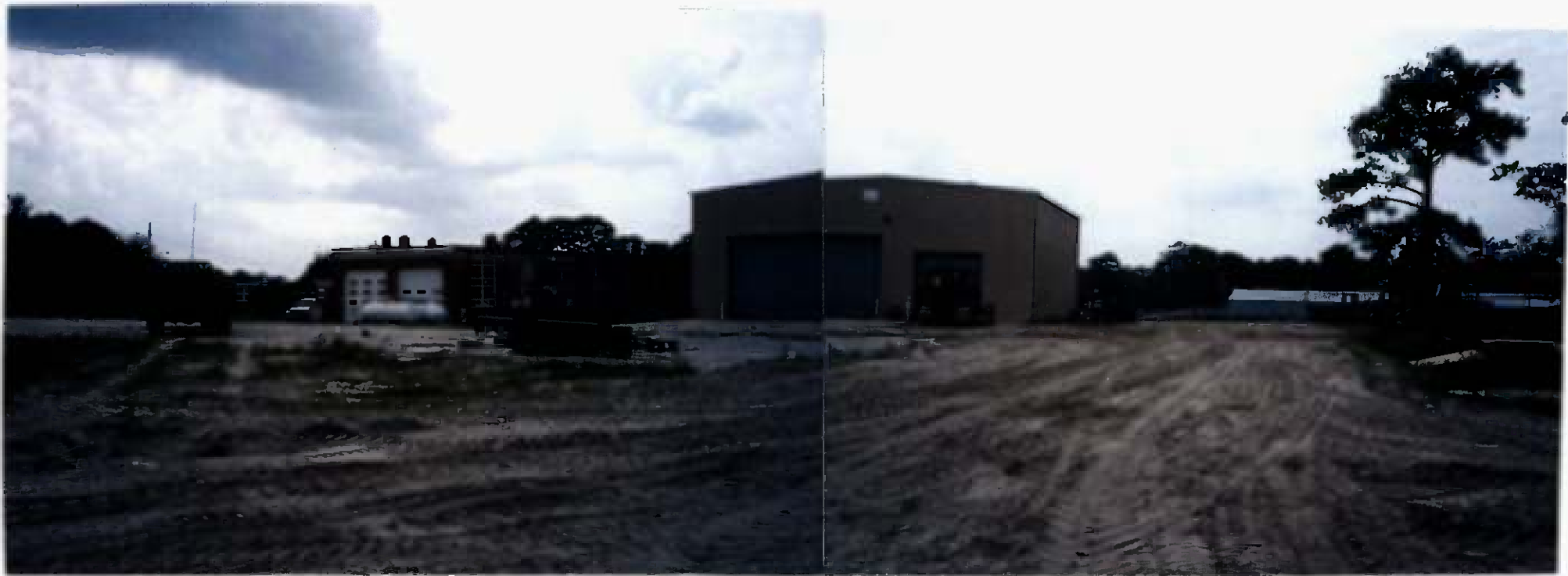
Site 91, Buildings BB-150 and BB-51, looking west.
