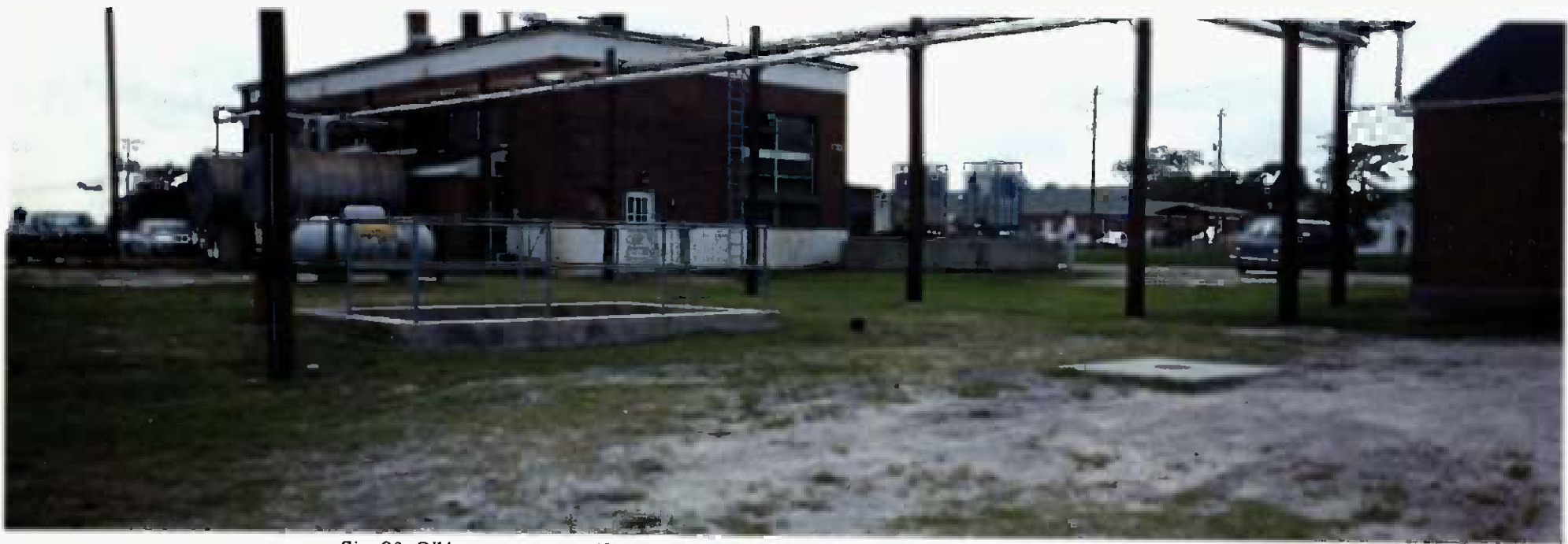
Site 90, Oil/water separator (foreground), UST excavation area, and Building BB-9 (background), looking southwest.
