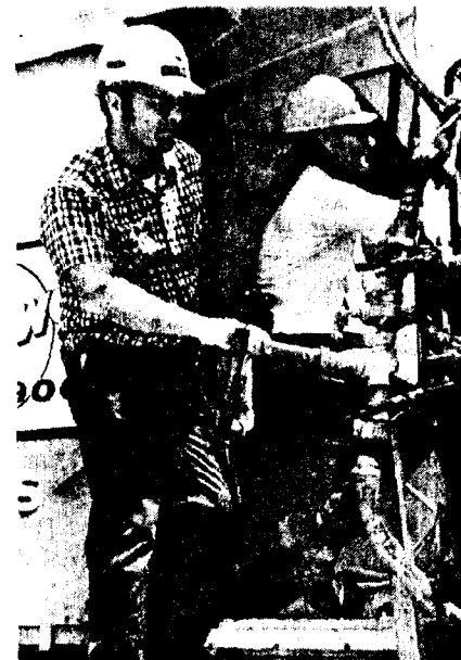
SLURRY SYSTEMS SUPERINTENDENT Bob Budgin and operator Dick Harris check alignment of slurry wall.
