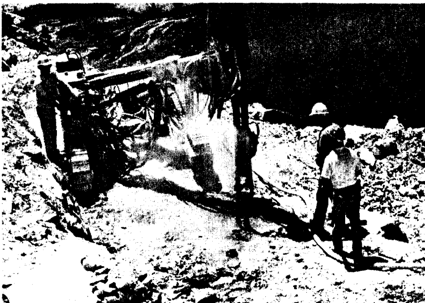
GARDNER-DENVER AIR-TRAC DRILL bores into a rock where a 1:1 bench is being cut for the earthfill dam's left abutment tie-in. About 8000 yds. of rock were shot from the bluff.
