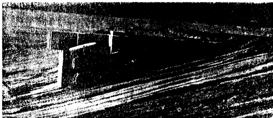
INSIDE of dike wall is bladed to 3:1 slope by a small International dozer working sand fill.
