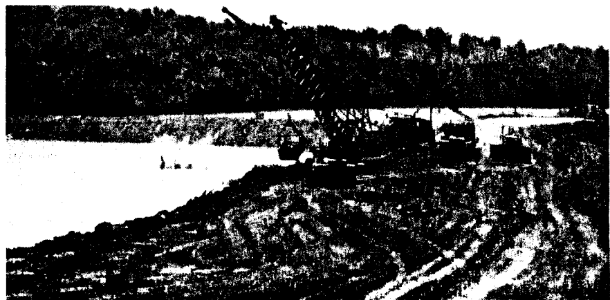
INJECTION RIG for slurry wall erection is seen from nearby Kaysinger Bluff at downstream closure dike (above). Below, Groves' Northwest dragline dumps a load of muck into a waiting Euclid bottom-dump while an American drops its bucket into water trapped between the closure dikes.
