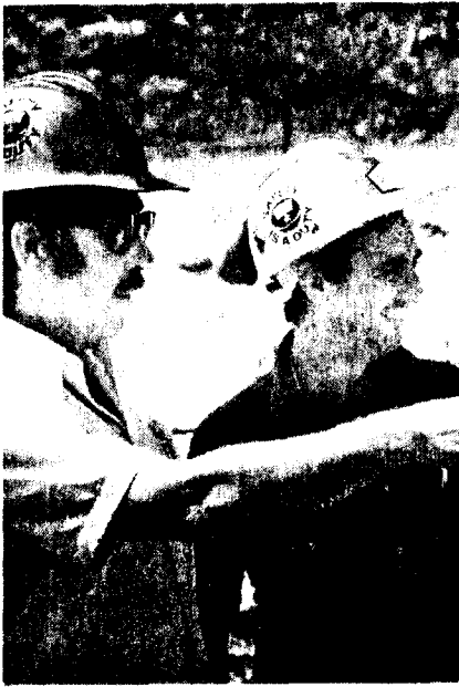
GENERAL SUPERINTENDENT Gerald Brister and project manager Charles Myers check dewatering.
