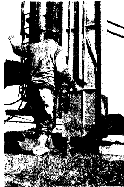
FOREMAN directs crane operator during positioning of injection beam that places 3.5-in.-thick slurry wall as it is driven into dike.
