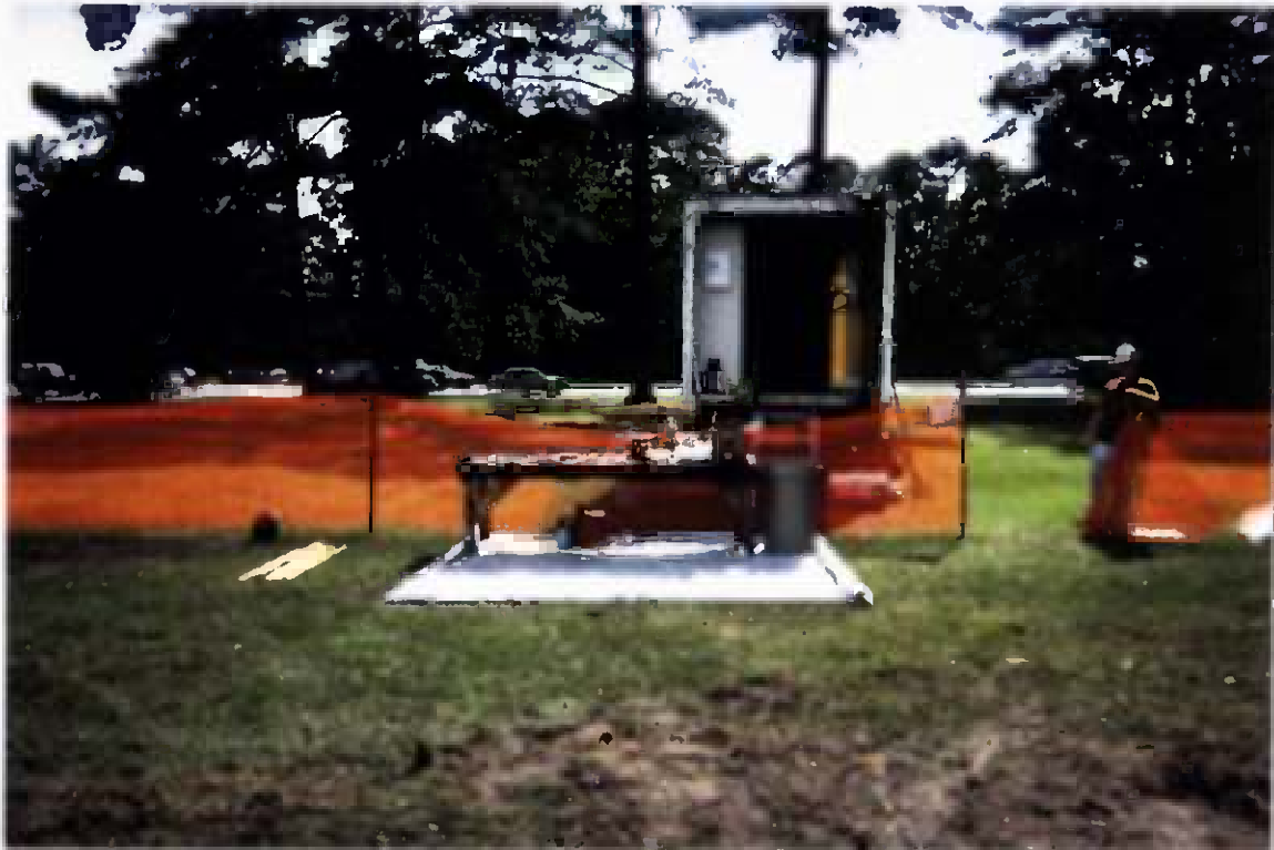
Project No. 16207 Contract No. N62470-93-D-3032 Delivery Order: 0023 Location : Area 1 Description: sampling equipment and decon area
