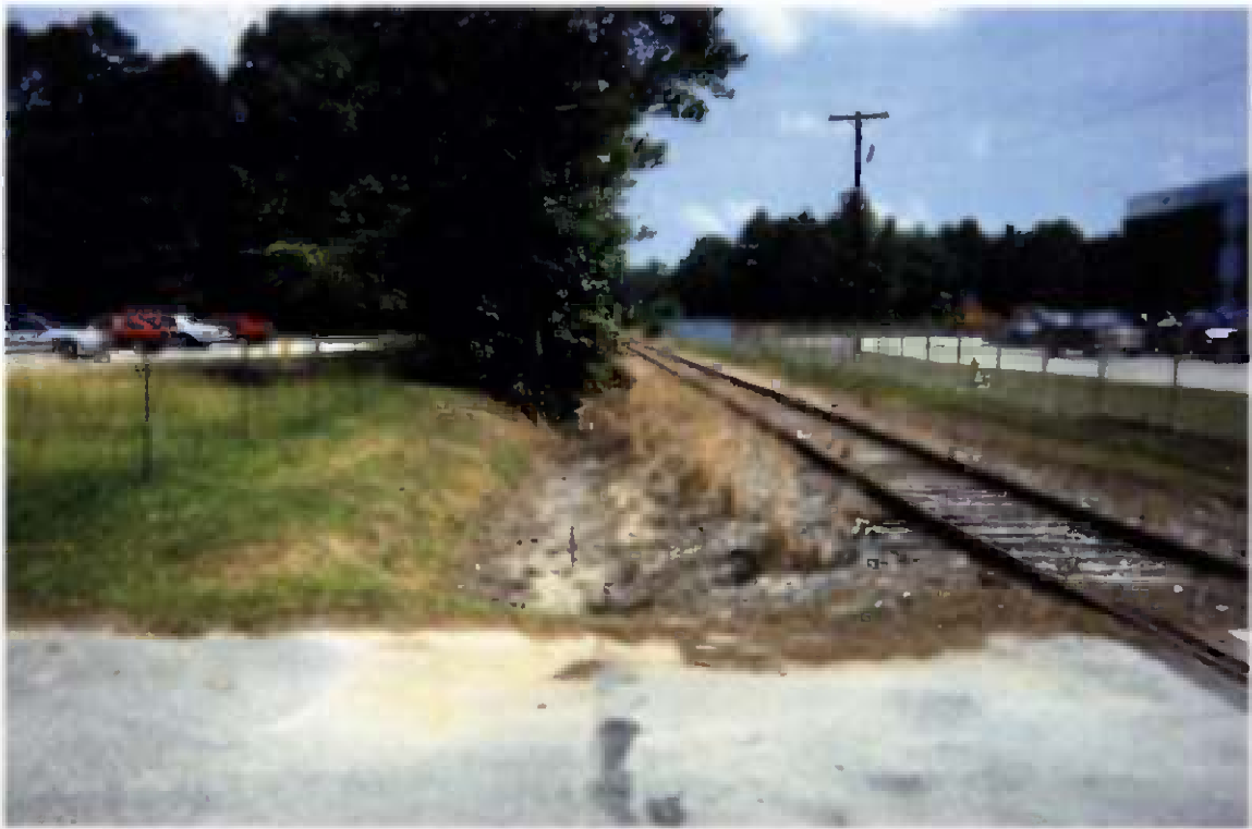
Project No. 16207 Contract No. N62470-93-D-3032 Delivery Order: 0023 Location : Area 1 Description: site prior to excavation
