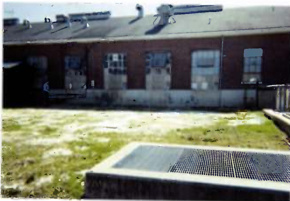
Photo # WP-1 Northern side of Building 25. The former UST system was located in the central portion of the photograph where very little grass is present. The grate in the foreground of the photograph is associated with underground steam lines.
