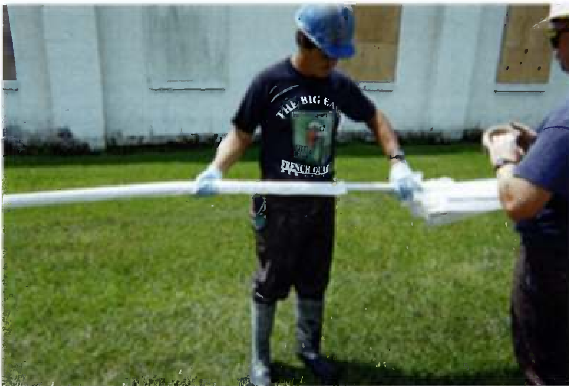
Photo # WP-5 Preparation of a temporary monitoring well, consisting of 1 inch diameter PVC and a synthetic filter sleeve. The filter, reduces the amount of fine grain material entering the well.
