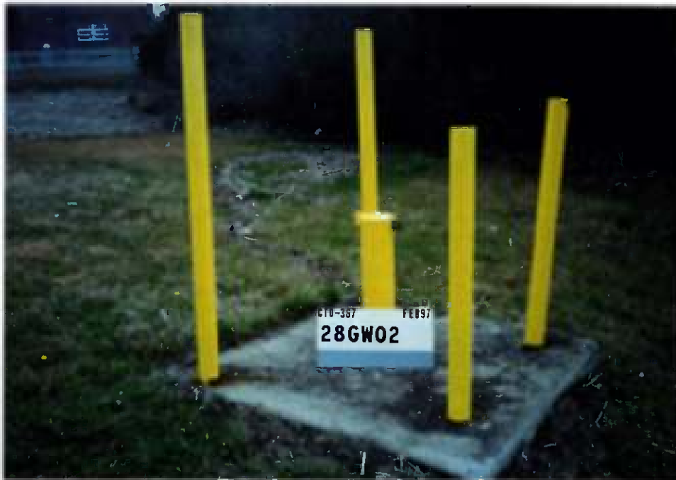
Figure 3-6 Peeling paint and rust were removed and two coats of weather resistant paint were then applied.
