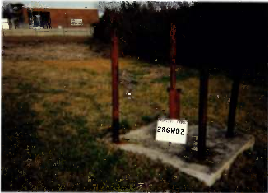
Figure 3-5 Shallow monitoring well 28-GW02 was installed during the 1984 Confirmation Study. The well had begun to exhibit signs of neglect and deterioration.
