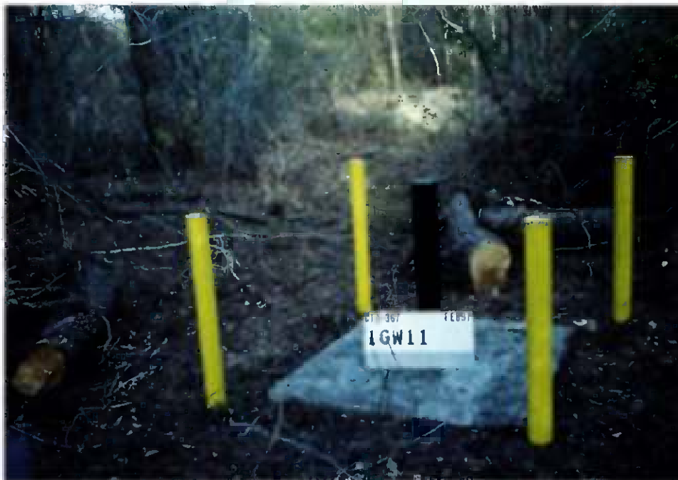
Figure 3-4 The fallen tree and debris were cleared and removed from 01-GW11.
